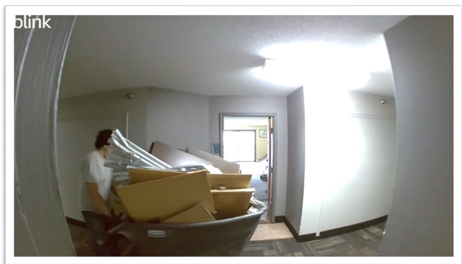
Carting uncovered demolition material in hallways after disturbance of suspect and presumed ACM.
